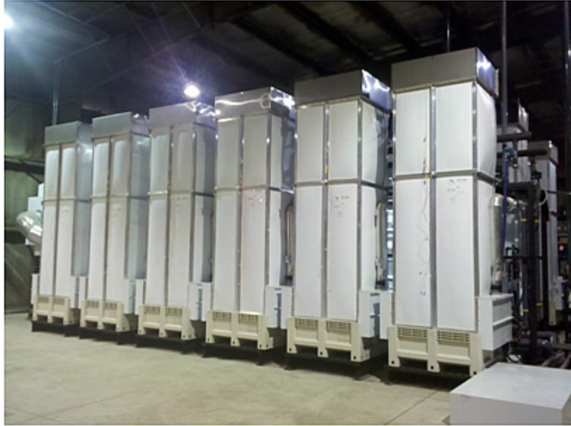
AltelaRain® 600 unit module and water treatment towers.
